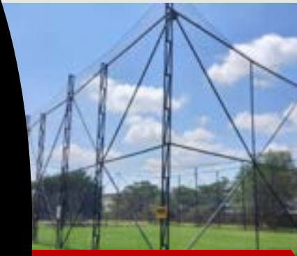
Drone cage & Drone Club. A first in the region
